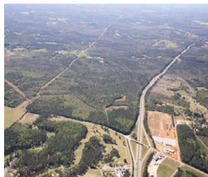
The new 463 acre Mid-Carolina Commerce Park at I-26 & Highway 773
