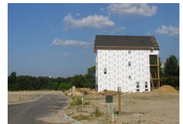
Home under construction at West Columbia's Village At Riverwalk
