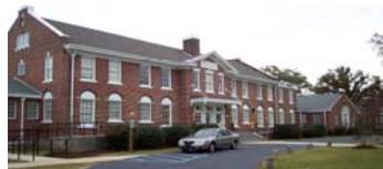
The renovated Newberry Hospital
