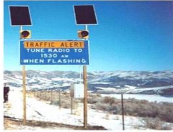
Rural ITS can warn drivers of changing driving conditions
