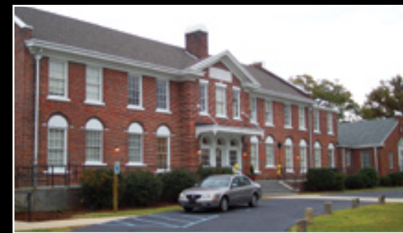
The completed $4.1 million old Newberry Hospital project
