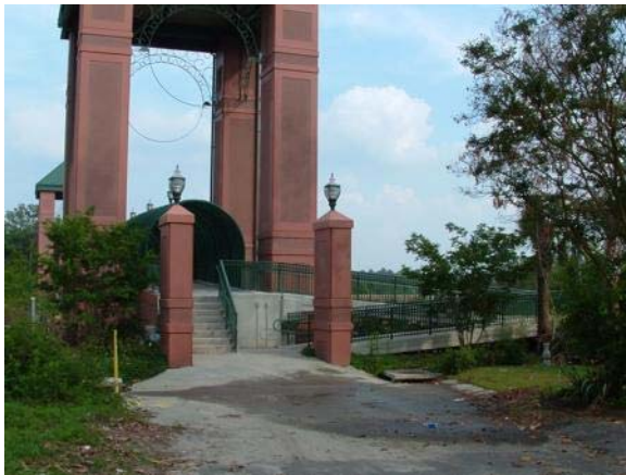
Western entrance to the James E. Clyburn Pedestrian Overpass
