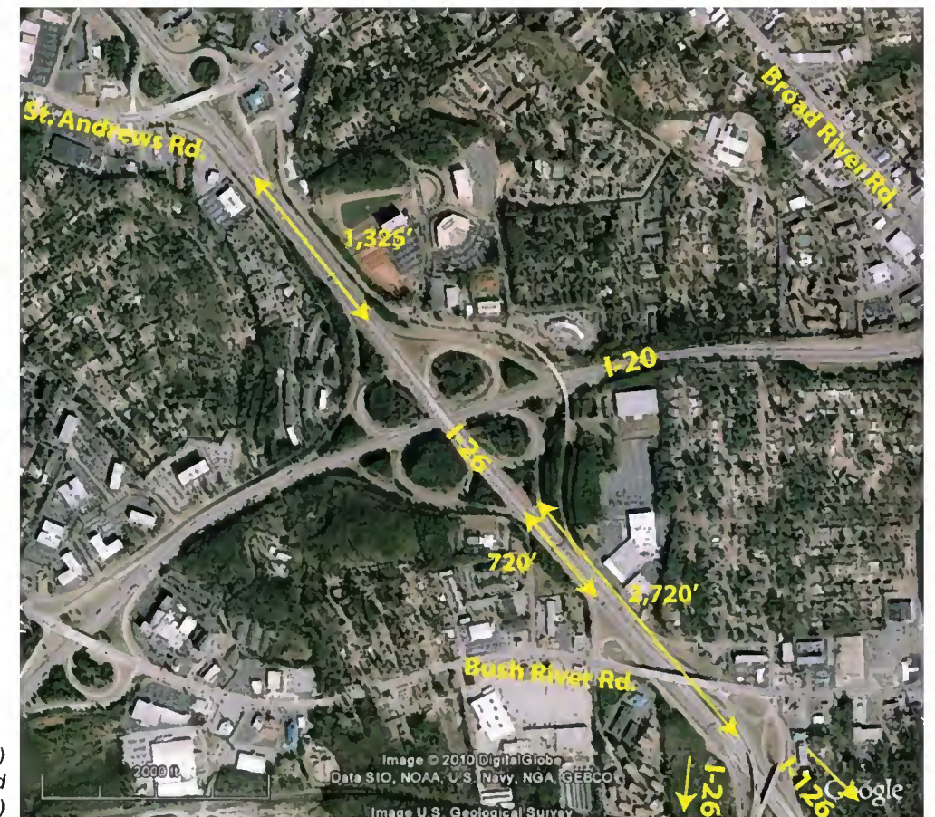
Figure 5.2 Interchanges at I-26 and I-20 (Top) Interchange at I-20 and Broad River Road (Bottom)
